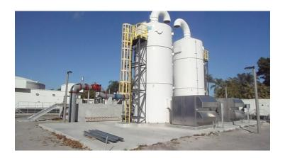
Two new degasifiers in the foreground and a new emergency generator on the back left, are just two of the ancillary items installed and ready to start service once the remainder of the construction is complete.
