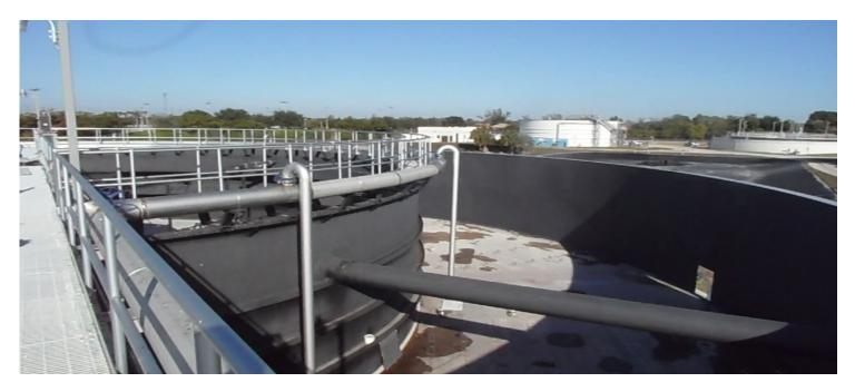
Above is the clarifier and digester section of a three-chambered 1.6 million gallon wastewater processing tank used for treating the inflow from the customers of the district. Once the process is complete the treated water will be injected 3,500 feet below ground as permitted for permanent disposal.
