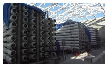
The construction progress photo above shows installation of three membrane "trains" and the high strength steel roof girders prior to the installation of the roof decking.
