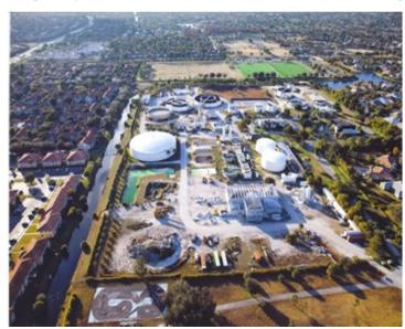
Aging facilities and improved water treatment processes were just two considerations taken into account when the decision to update our facilities was made. The current "Lime Softening" method of treating our water supply will soon be phased out and replaced by a state of the art 6.5 million gallon per day Membrane Filtration Treatment Plant. The pictures highlight the design and progress of the work.
